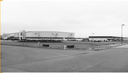
Fay-Penn's Multi-Tenant Facilities Fayette Business Park.
