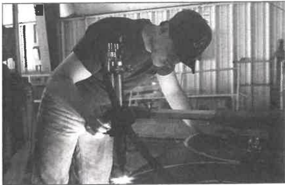
An employee cuts steel plating at Ceramic Fiber Technologies' new facility in North Union Township.
