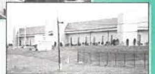
Nu-Metrics' beautiful, new world headquarters building is one of Fayette County's newest landmarks.
