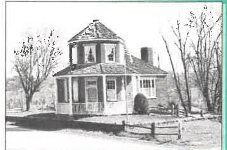
One of only two remaining toll houses along the National Road in PA, Searight's Toll House will receive much needed repairs.
